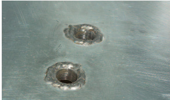
Picture 35. Fuel pipe bosses welded from inside the tank.
